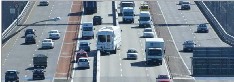
Quickchange® Moveable Barrier (QMB™) is designed to cost effectively increase capacity and reduce congestion by making more efficient use of new or existing roadways. Applications include high volume highways where additional right-of-way may not be available, where environmental concerns may exist, or where the lack of funding may slow or inhibit support for new construction.
